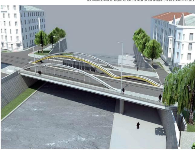
different moments to avoid the interruption of the traffic, one carriageway per time: firstly one way of the existing bridge has been demolished, then the new structures assembled on the ground and lastly launched in its final position with the aid of a launching nose.
